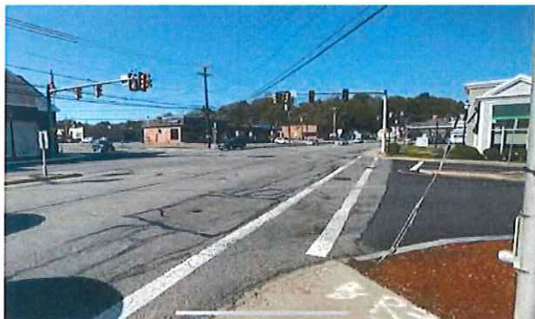
Pictured: Crosswalk across Plaza Driveway where crosswalk width does not meet ADA compliance and no detectable warning pads of APS pushbuttons exists.
